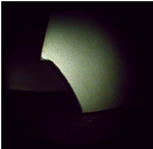
This view is showing a stage 1-R rotor blade tip failure.
