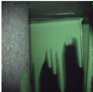
This view is showing a stage 17-S vane being tested remotely using fluorescent dye penetrant.
