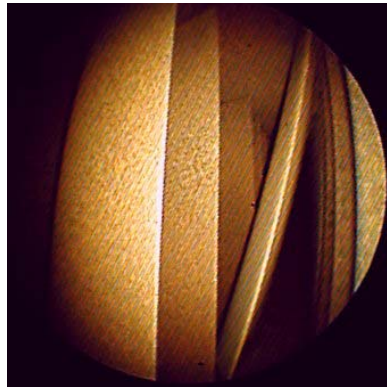
This view is showing a stage 17-S vane failure.
